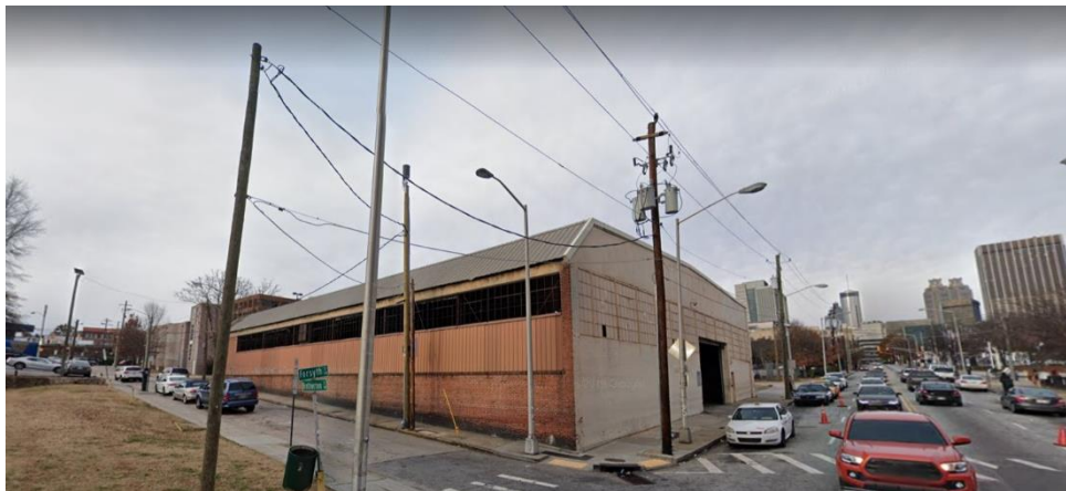
Figure 36. Vehicle flow in Route 3 in Mechanicsville
