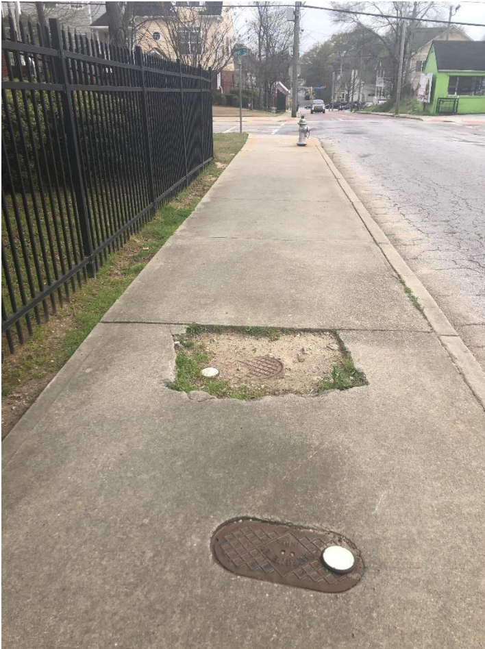
Figure 16. Sidewalk in Mechanicsville
