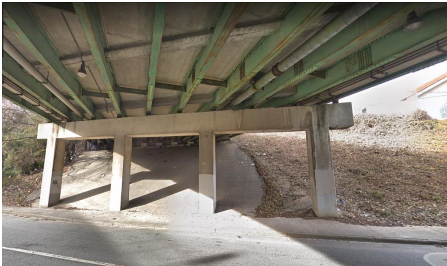
Figure 41. Underpass during Route 3
