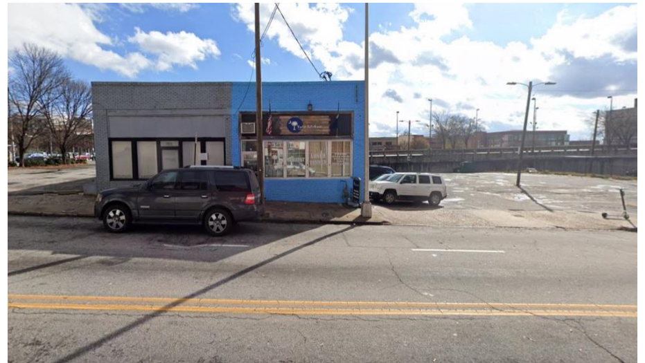
Figure 38. Abandoned building next to Kelz Kitchen
