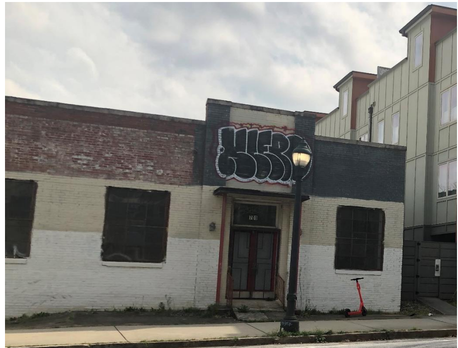
Figure 48. Abandoned building in Inman Park
