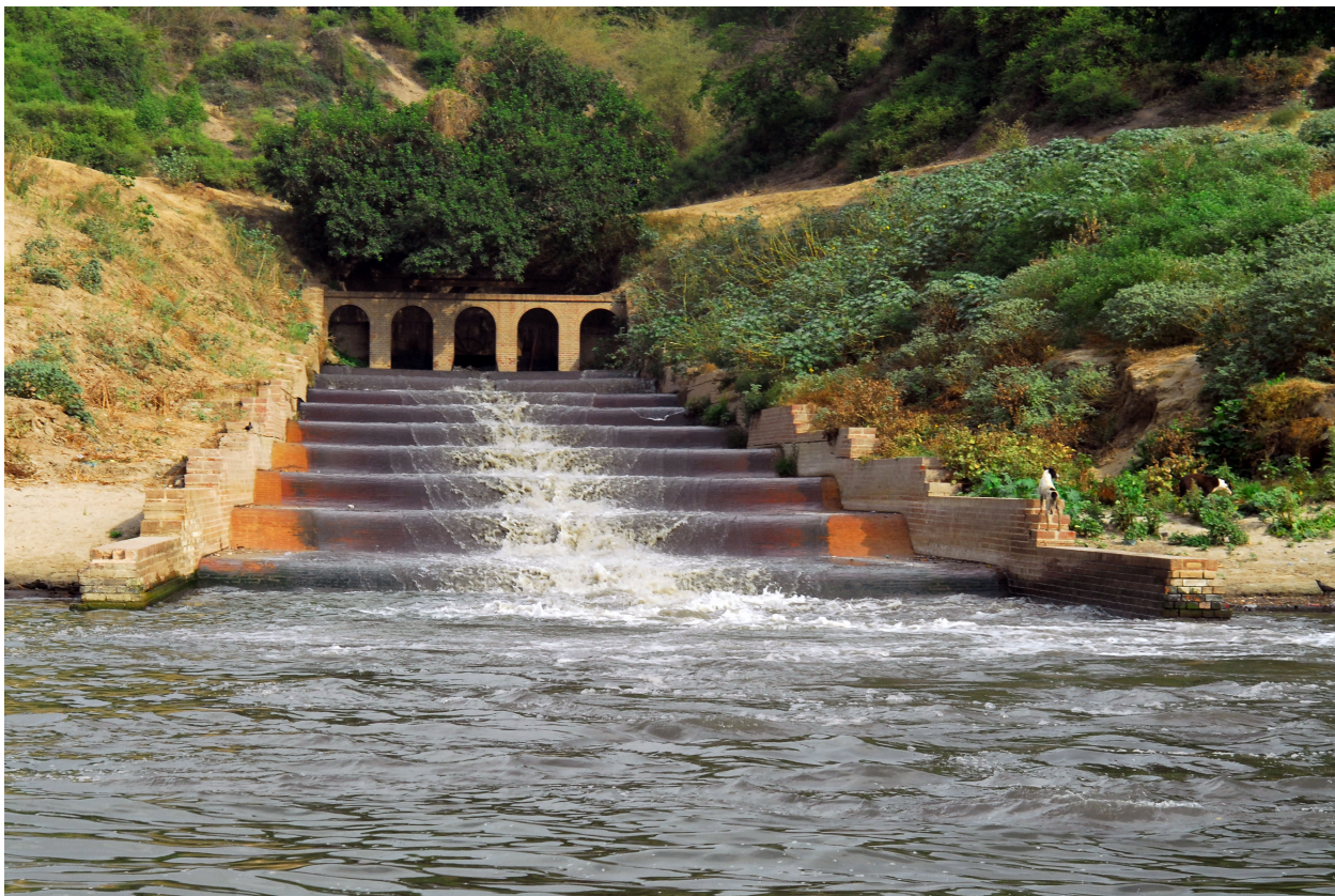
Figure 13: Main Trunk Sewer Outfall Varanasi, India
