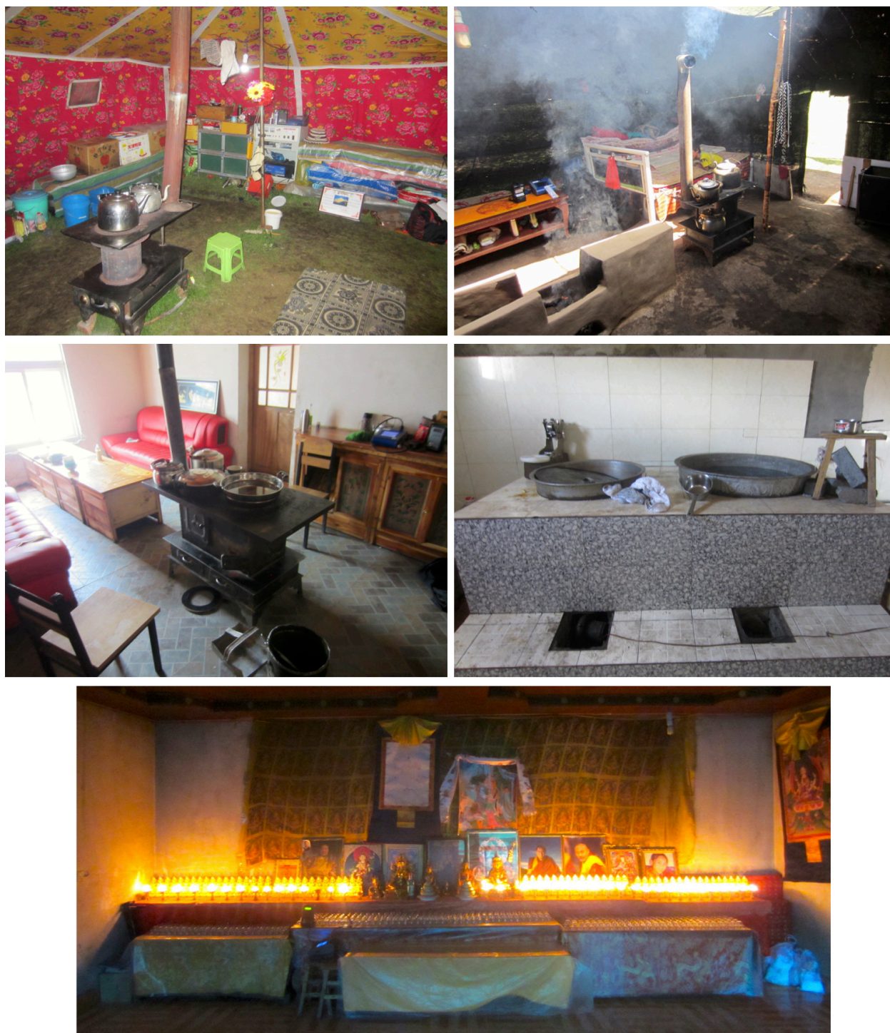
Figure 3. Various combustion sources where HAP was measured: top left , improved stove in a tarp tent; top right , traditional adobe stove beside an improved stove in yak hair tent (note how stovepipe terminates inside tent); middle left , teachers' kitchen; middle right , different type of improved stove in cafeteria kitchen; bottom , yak butter candles in a prayer room
