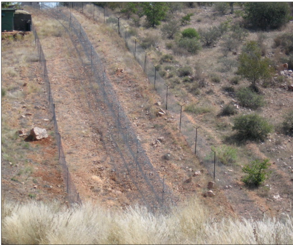
Fig. 7 Part of the three-tier fence on the South African side of the border with Zimbabwe. The middle row is the one that once was electrified. [Photo by Author, 2010]
