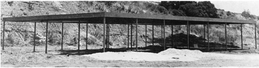
Figure 9: Photograph of Case Study House 1950's steel frame. Raphael Soriano, "Case Study House 1950," Arts and Architecture , September 1950, 36.
