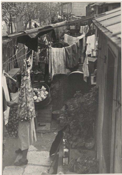
Figure 2: “Cluttered backyards, with clotheslines and poorly made fences drawing the boundaries between neighbors,” Los Angeles. From Poor Housing Conditions in Los Angeles Scrapbook (1938).
