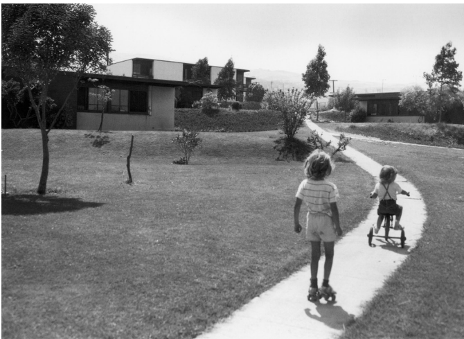
Figure 14: “Channel Heights Housing, 1941-1942” (San Pedro, Ca.). Richard Neutra, architect. Architectural Plans and Section, The Avery Library and The Graduate School of Architecture, Planning and Preservation, Columbia University, New York, New York.
