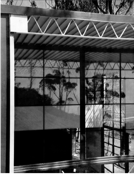
Figure 11: Detail of Case Study House 1949. John Entenza and Charles Eames, “Case Study House 1949” Arts and Architecture , December 1949, 34.
