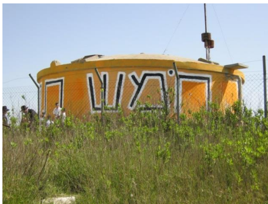
Figure 16 Water tower at Chomesh
