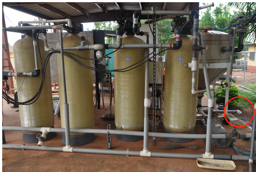
Figure 3: Raw water sample site at Kintampo Municipal Hospital.
