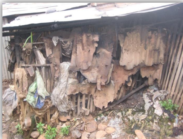
Photo Set 1: Kitchens Monitored for Indoor Air Pollution. Kitchens were a separate unit from the household and constructed from sheet metal, mud, and other materials
