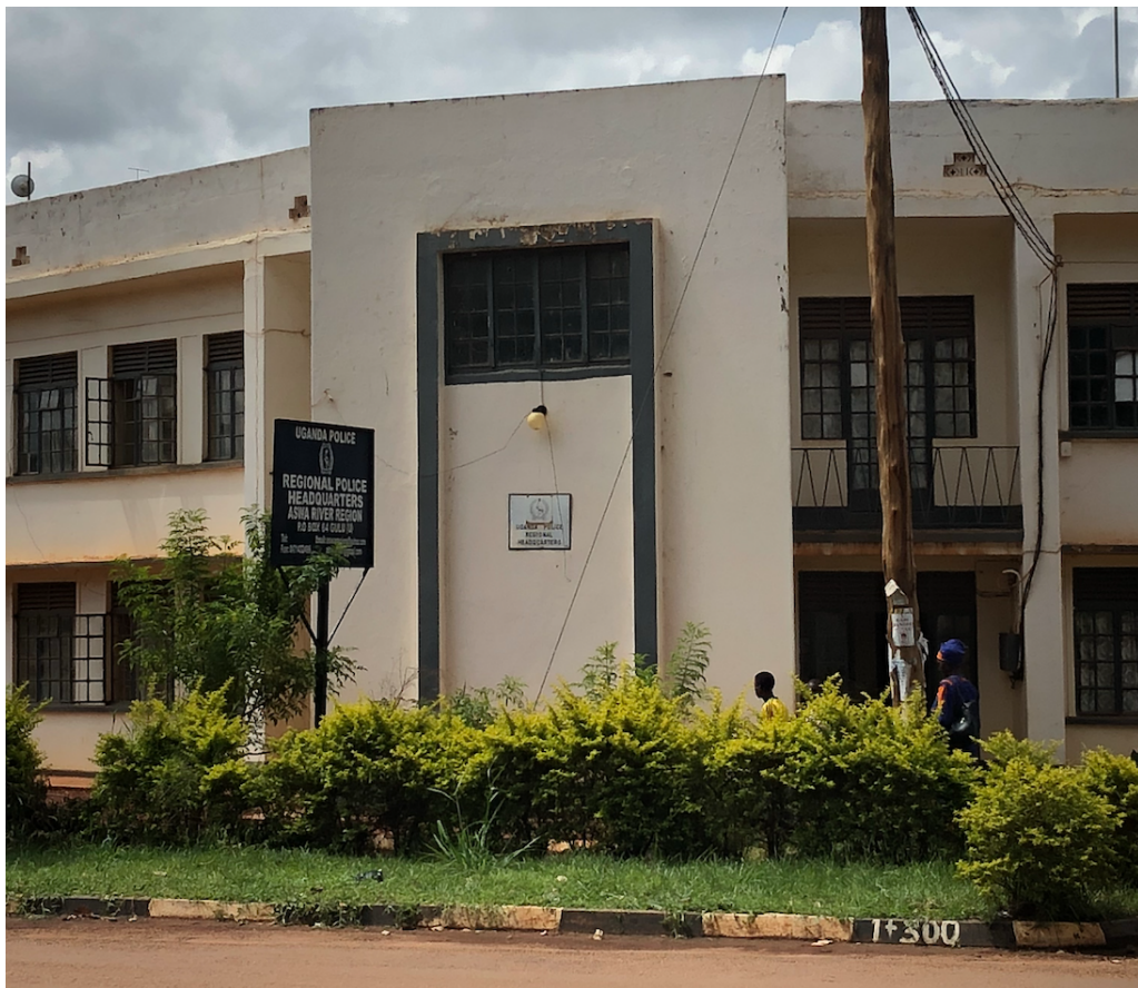
Figure 7.9: Uganda Police Regional Headquarters, Gulu.
