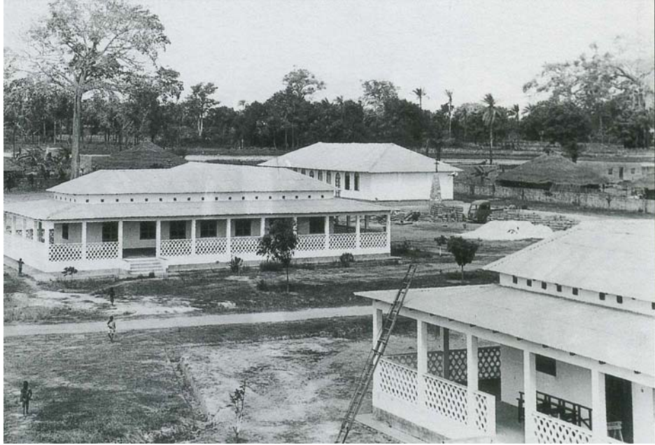
Construction of the PIME Mission facilities in Susana. Nuns' house in background, priests' house in foreground, and the first church (later dismantled) in the far background (Gheddo 1999).
