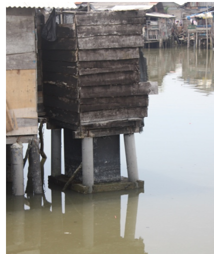
Figure 13. Sanitation System Type 3 - Typical Installation
