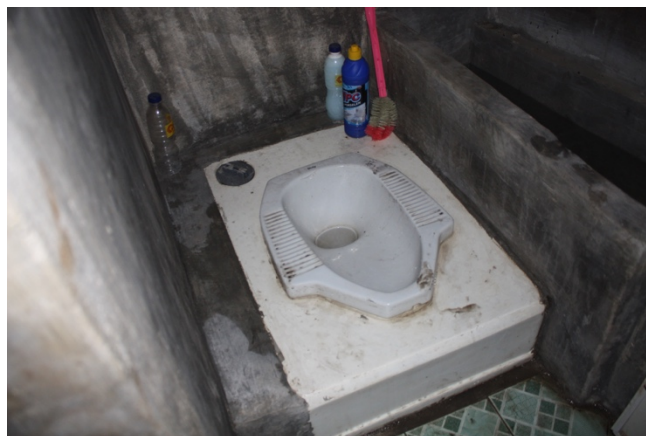
Figure 16. Sanitation System Type 5 - Typical Squat Plate
