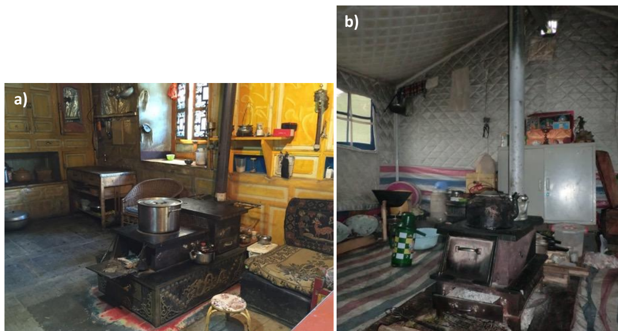
Figure A1. Traditional Tibetan style cast-iron stoves with chimneys from surveyed households. a) stove in a traditional Tibetan house from the agricultural village, b) stove in a tent from the nomadic village.
