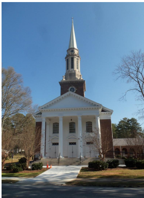
Figure 6. Formerly Audubon Forest United Methodist Church, this building is now used by Hoosier Memorial United Methodist Church. (photo by author)
