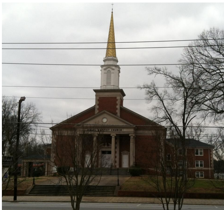
Figure 2. The sanctuary of Kirkwood Baptist Church, built in 1953, is now owned by Israel Baptist Church. (photo by author)
