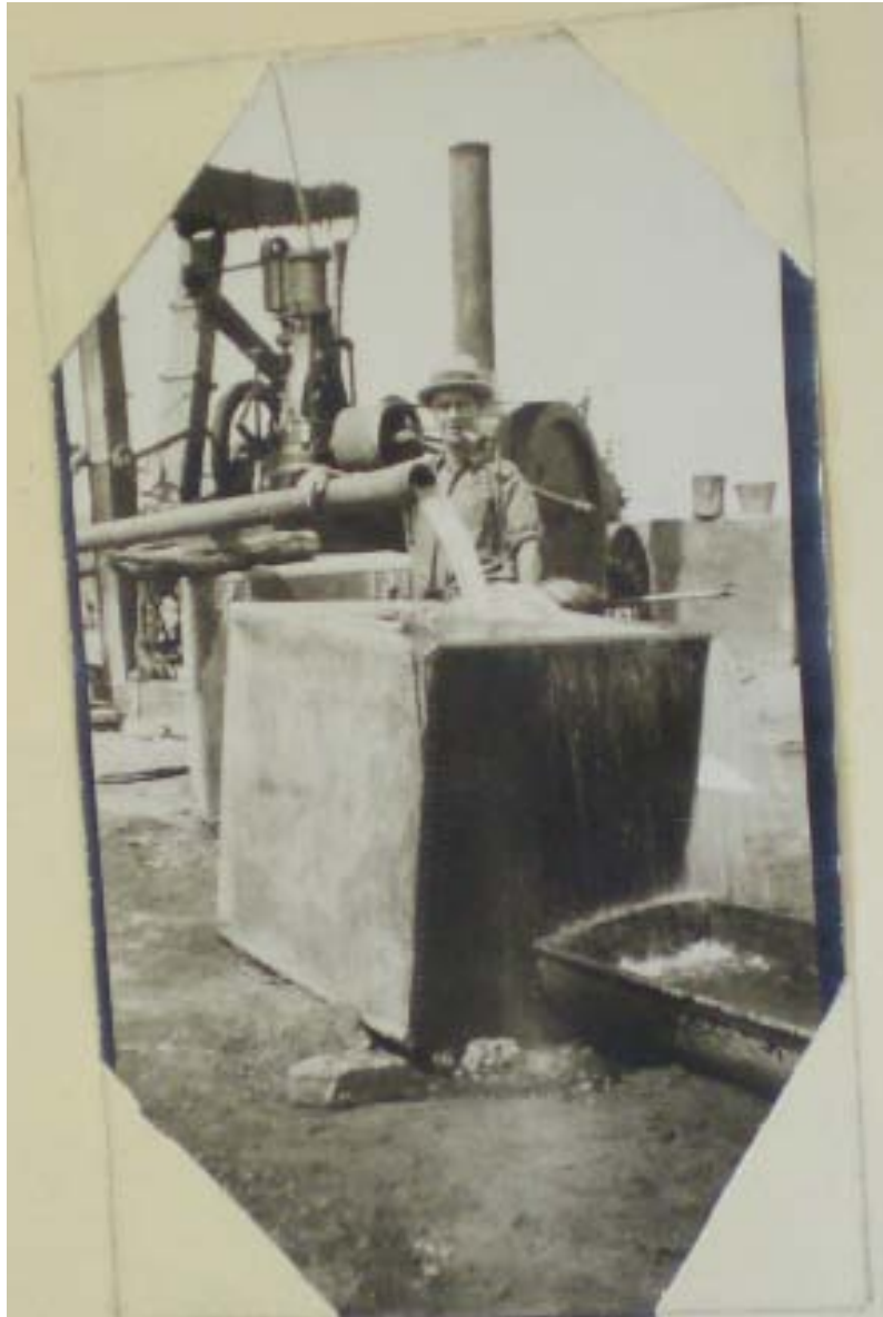
Figure 3: Second Borehole in Epukiro, 1923 201
