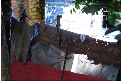
Figure 23: Layers of new construction materials for the poorest families in Joya de Cerén.
