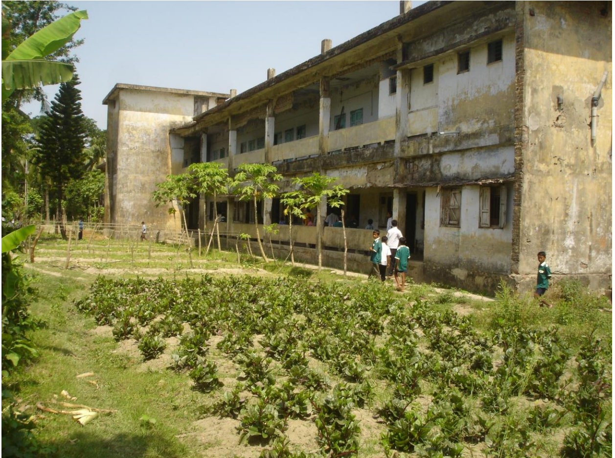
Photograph 2.3: The original orphanage building, built after the 1970 cyclone to house the many children left without families.
