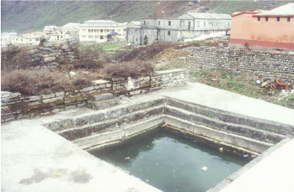
Figure II.19. Hams Kund, looking southwest.
