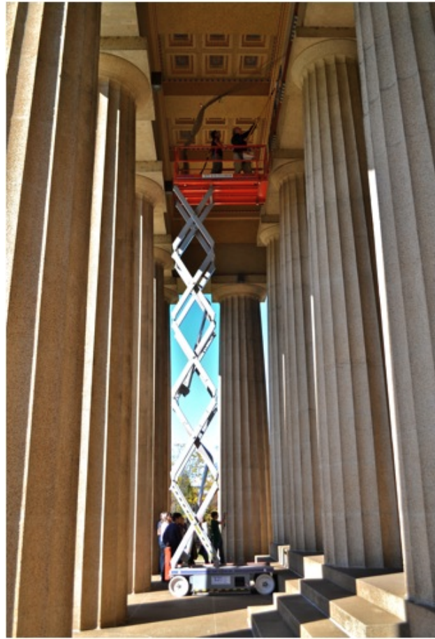
Figure 3.22 A specialty lift was used to reach the frieze course (Image: Nashville Tennessean (left) and Jiang (right))
