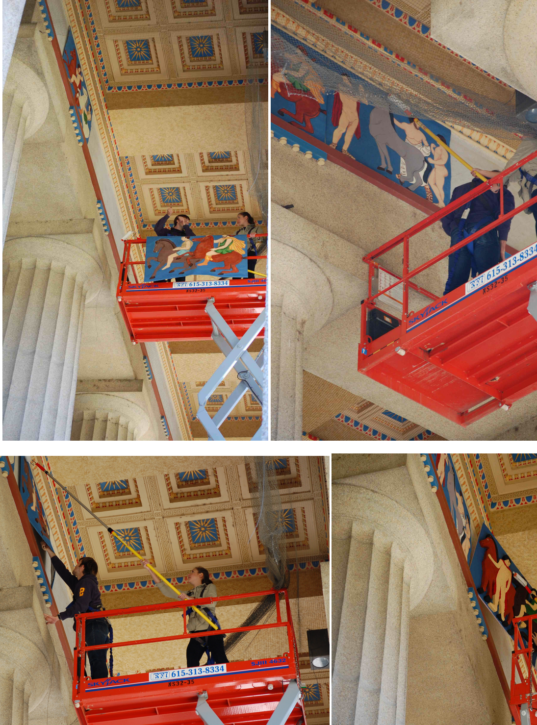
Figure 3.23 The frieze panels were positioned and installed using velcro and a paint roller. The same method was used for the relief panel. (All Images: Cupello)
