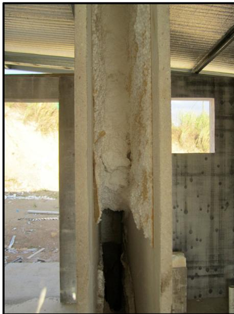
*Single family home interior wall with Styrofoam insulation.*
