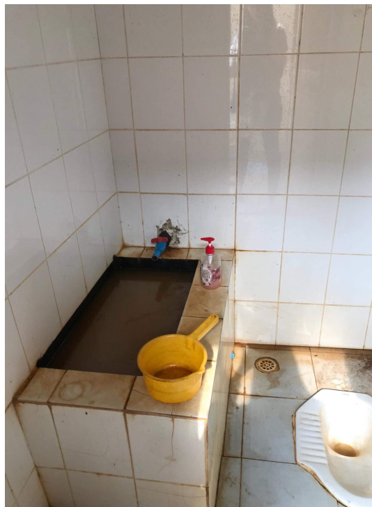
Figure 1. A toilet in health center B
