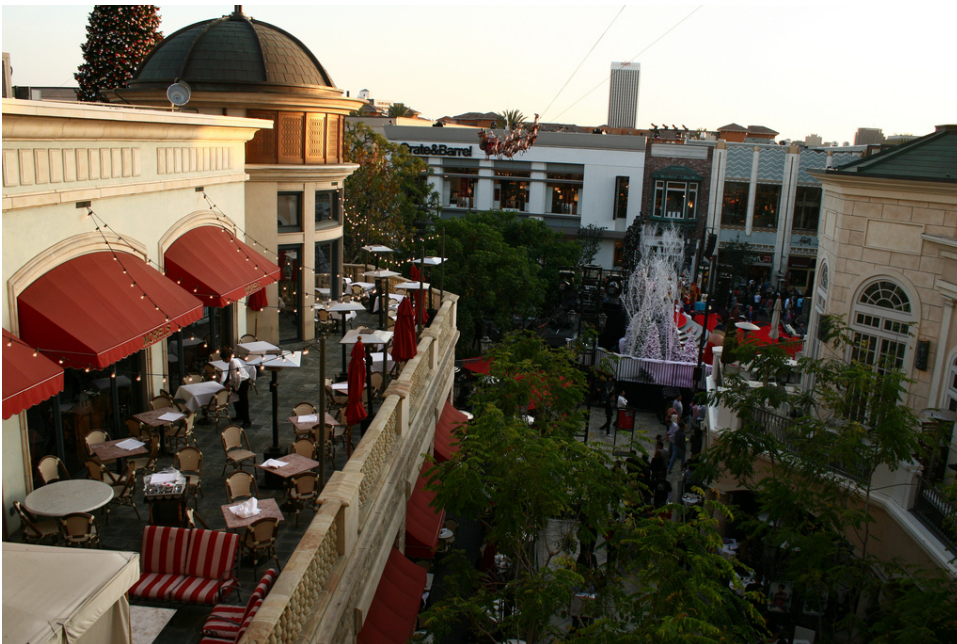
Figure 26. The Grove, a mixed-use development in Los Angeles completed in 2002, served as inspiration for Avalon. Source: Prayitno, Flickr, 2009. Attribution 2.0 Generic (CC by 2.0).
