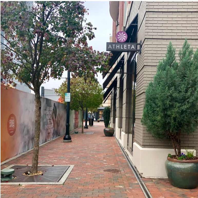
Figure 18. A rubber and metal expansion joint runs along the sidewalk and lines the edge of buildings in the retail district. Source: Matthew Heldman, 2018.
