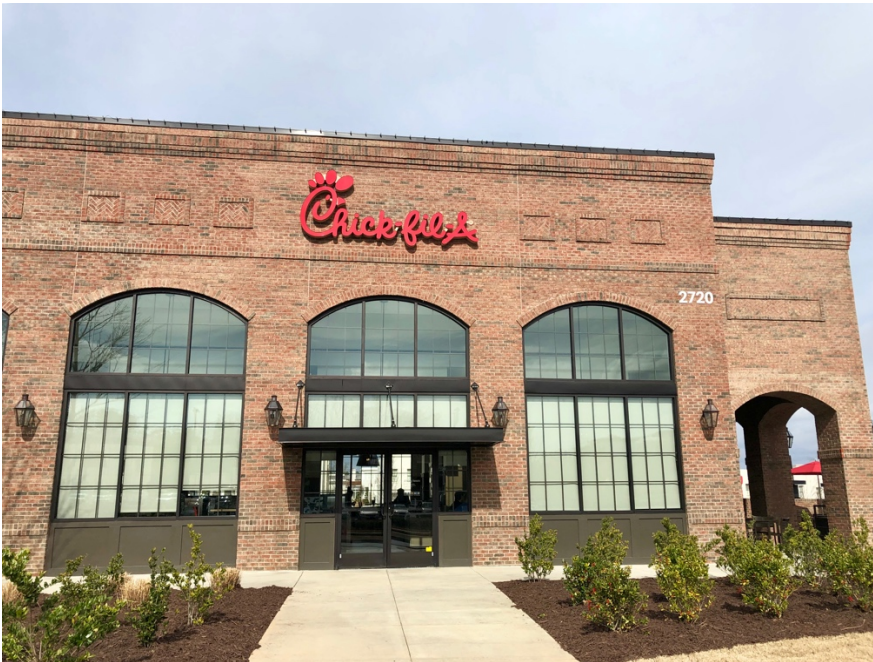
Figure 32. A standalone Chick-fil-A on the edge of the Avalon property, off of Old Milton Pkwy. The structure, which does not look like a typical Chick-fil-A, was constructed to mimic a repurposed industrial warehouse with brick and large, arched glass windows—a trendy aesthetic associated with millennial’s movement back to urban areas. A closer look will show expansion joints running vertically aligned with the left edge of each window.
