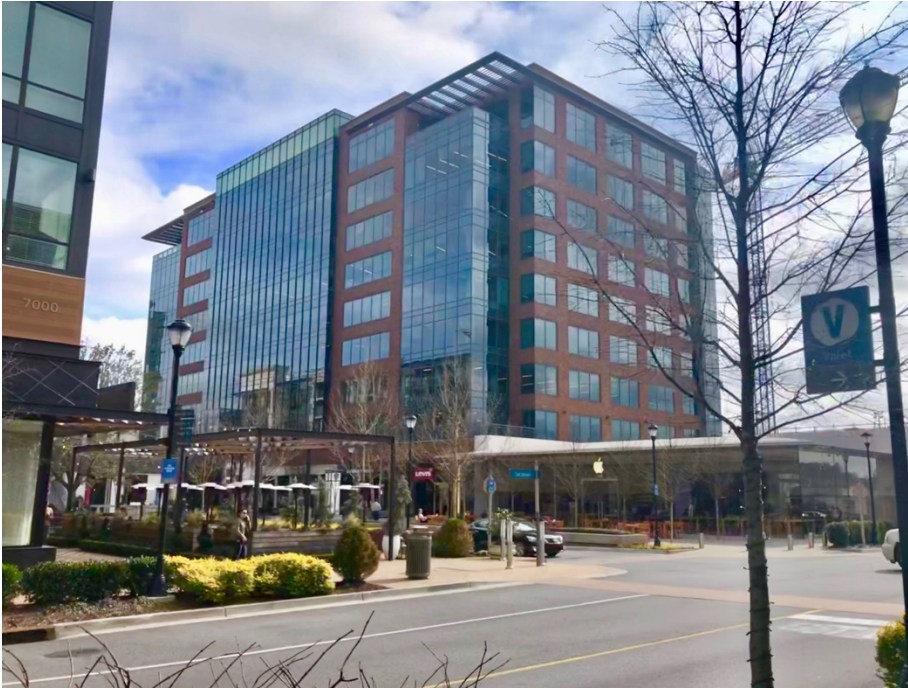
Figure 31. Building 8000, an office tower at Avalon that has street-level retail. Source: Matthew Heldman, 2019.
