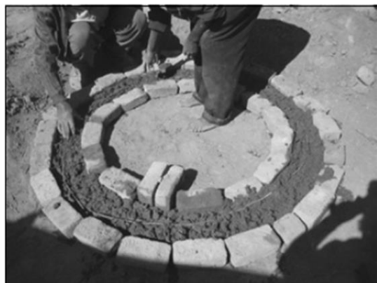
Figure 5: Making an arborloo ring beam (Morgan 2007a)
