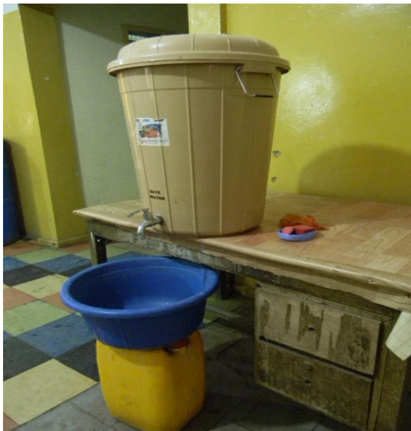
Figure 15: A veronica bucket used for water storage and hand washing within hospital wards.
