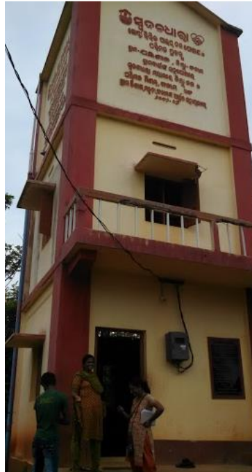
Figure B1. Community water tower with reservoir above, and community meeting room below.
