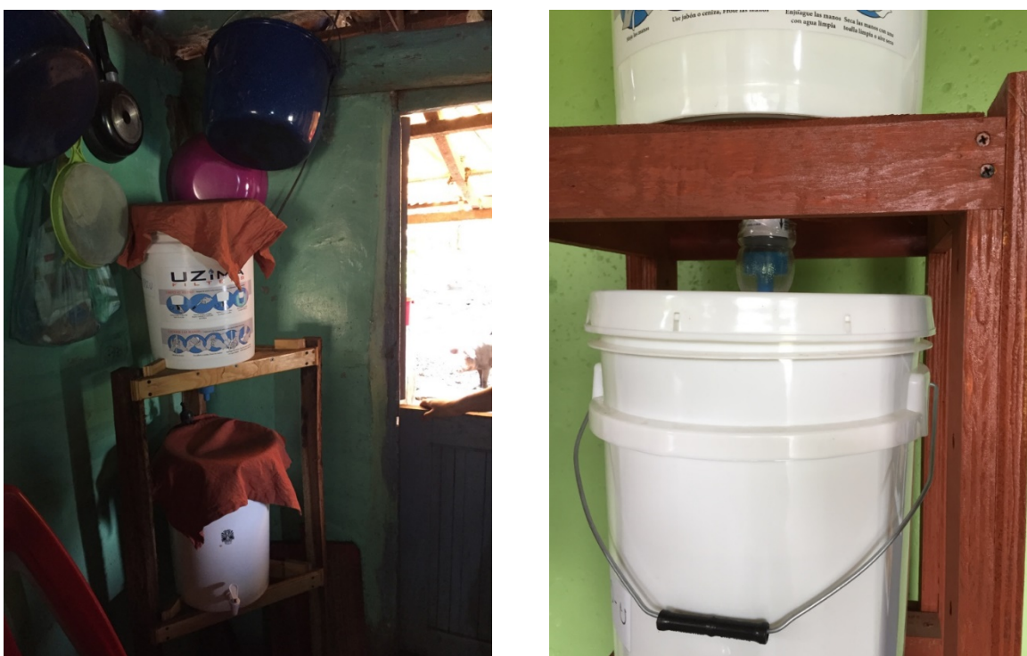
Figure 5 Techniques to prevent contamination of filters on wooden stands in project households in the midline evaluation of a hollow fiber membrane filtration program in the Agalta Valley, Honduras, January-July 2016 (Reproduced with permission from Sera Global Health Practice)
