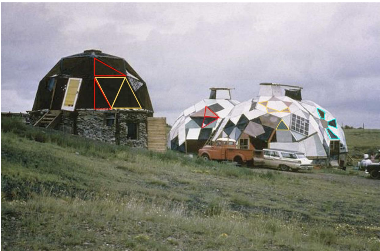
Figure 2.3: The Hole (L) and The Complex (R) in 1967. The Hole is built into the side of a hill. The base is not a dome shape; it looks instead like the base of a stone column. The top part of The Hole is similar to Fuller's geodesic dome design, composed entirely of triangularly shaped pieces, including both right triangles and equilateral triangles. Some of these triangles are indicated in color; the red outlines indicate right triangles, while the yellow outlines indicate equilateral triangles. The Complex's structure experiments with the geodesic dome structure in a different way. The Complex is composed of three interconnected geodesic domes. A part of the structure visible to the viewer also uses elongated trapezoid shapes, indicated in blue, that encircle a pentagonal shape.
