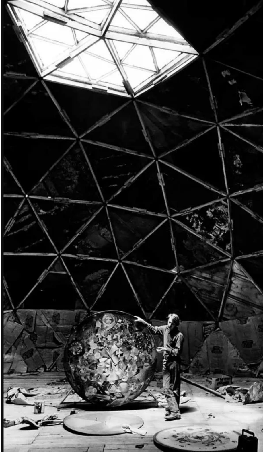
Figure 2.7: Clark Richert poses with The Ultimate Painting in the Theater Dome. The image reveals quite how dark some of the domes' interiors could be. The wood flooring that does sit directly below the skylight is cast into darkness. Drop City did have electricity, and so it is possible that some of the domes used electric lights to help light the interiors. The skylights and other windows were also intended to create more light inside the structures.
