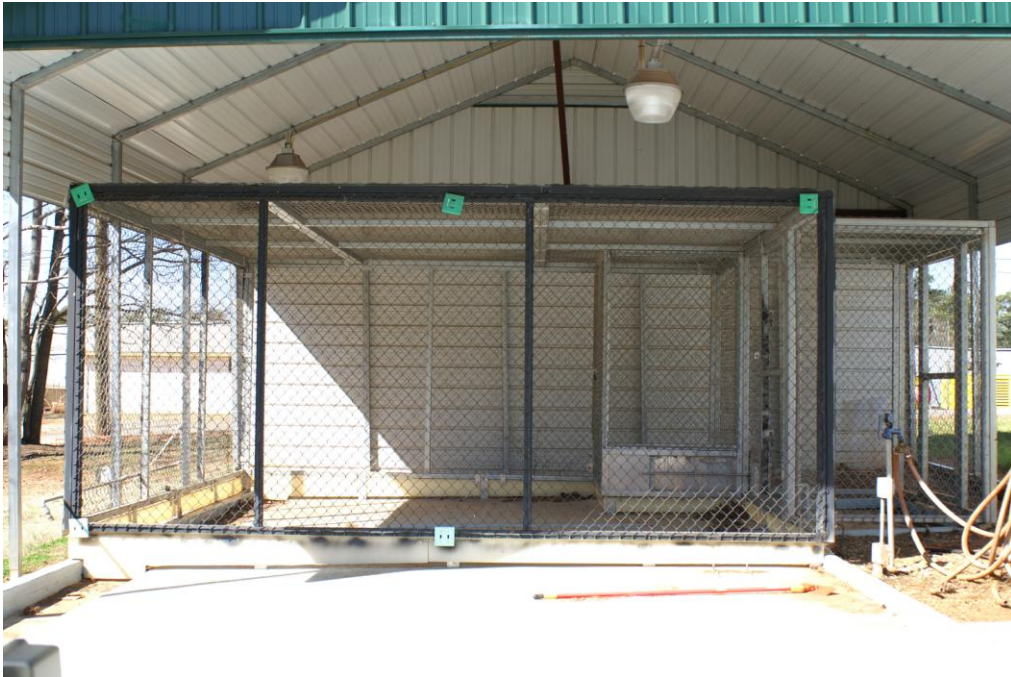
Figure 1. The testing facility (view from the east side of the facility).
