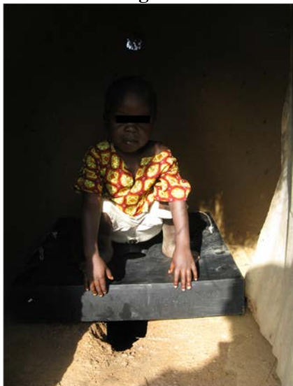
Image 13: The #2 LTM covers the latrine's larger hole
