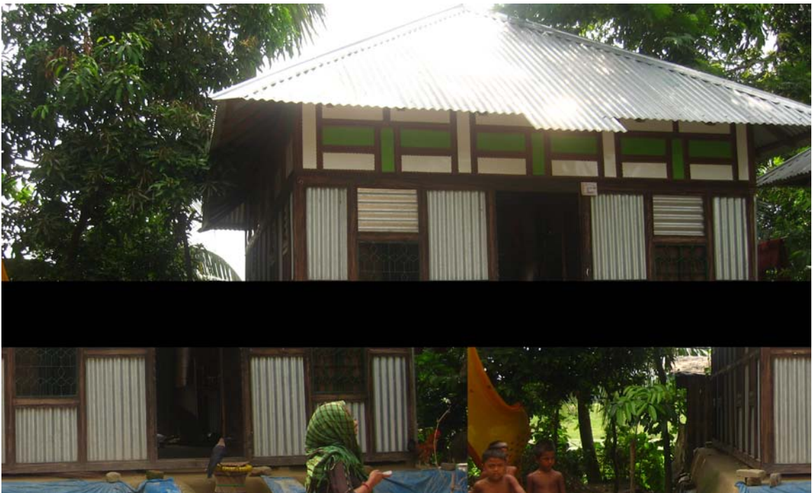
Figure 5. Housing structure built from metal sheets with firm mud foundation
