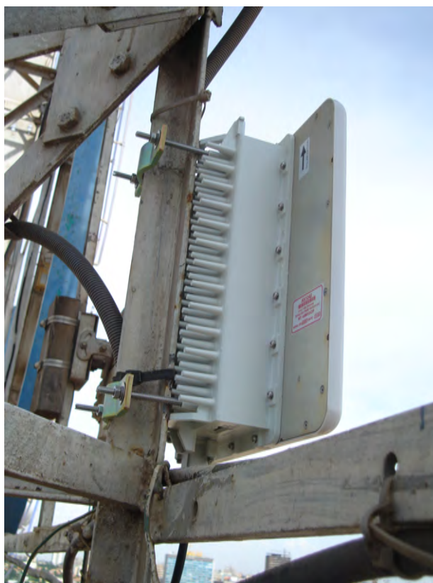
Fig. 77. Wireless transmitter used by Internet Technologies Angola, ISP of the Trienal de Luanda. Broadcasts from atop the BPC building in downtown Luanda and is received by a satellite that communicates directly with Brazilian hosts.
