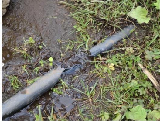
Figure 9: Plastic covering wrapped around the Bushokoro Pipeline, Bisate, Rwanda
