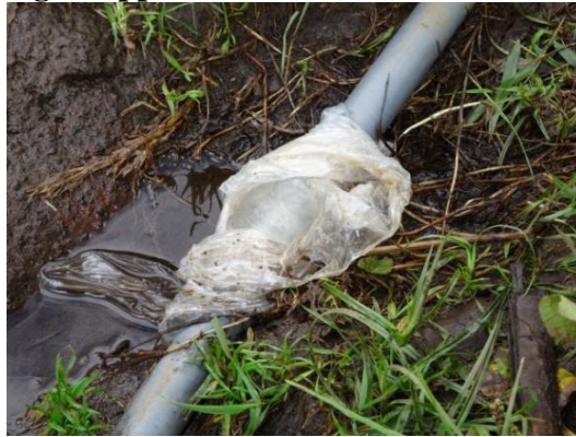
Figure 9: Plastic covering wrapped around the Bushokoro Pipeline, Bisate, Rwanda
