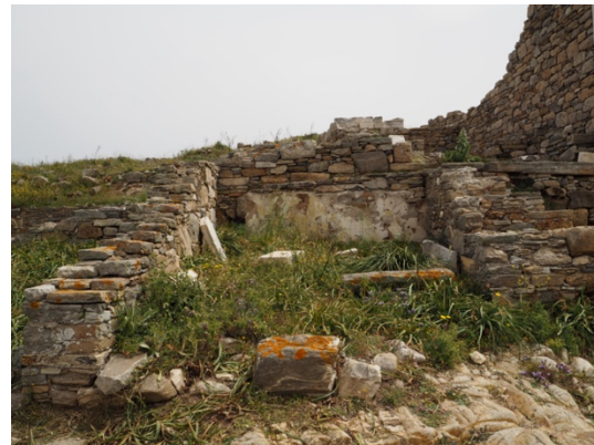
Current state, view from the west.
