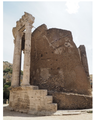
Current state, view from the northwest. Photo: A. Eckhardt
