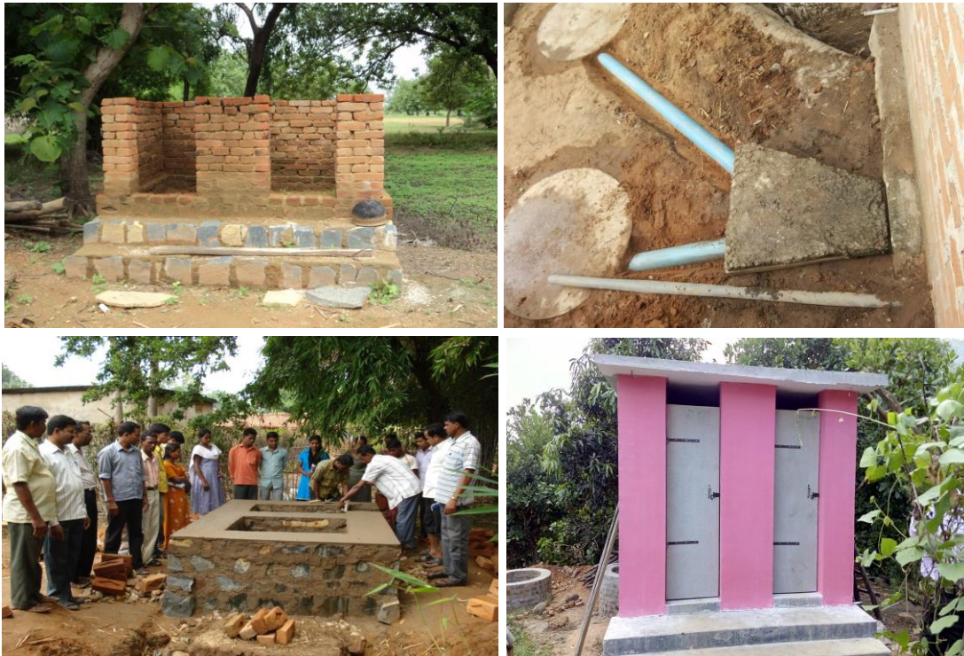
Figure 2: Photographs of the construction of the household sanitary unit
