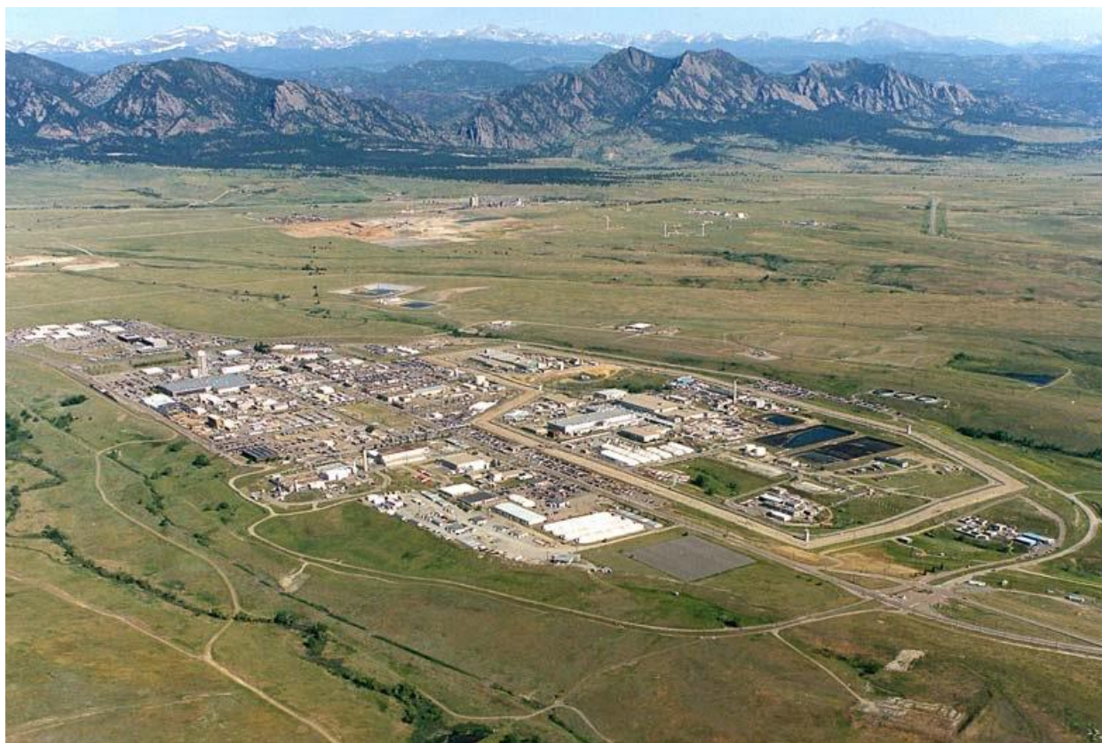
Figure 6: An aerial Photo of the Rocky Flats Site taken in 2001. The buildings depicted make up the “Industrial Zone” as it was before most of the buildings were demolished. 124
