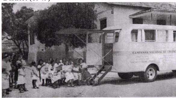
Figure 3.10: DNCr/CNC mobile post in the Federal District (1949)
