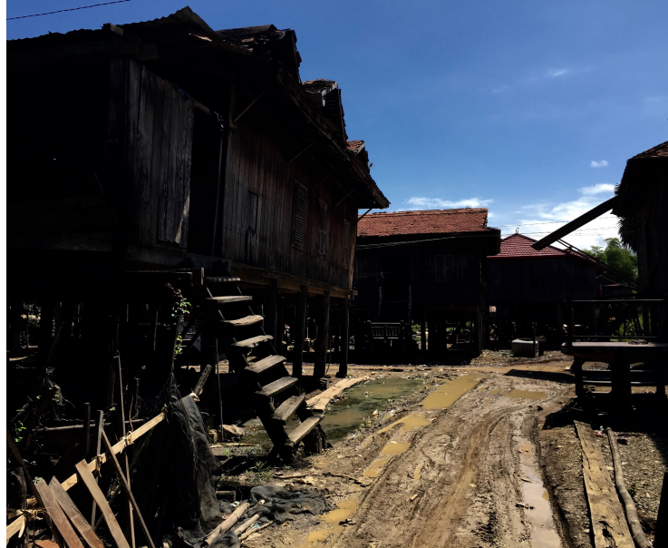
A participant shows the outside of her home. The stairs are especially slippery when it rains. Difficulties associated with stairs could be diminished by use of ramps with low slope gradients, or with the addition of sturdy wooden handrails where construction of ramps is less feasible.
