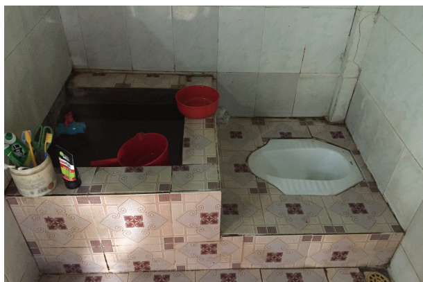
Pictured is a specially constructed low-to-the-ground toilet and bath, modified for a participant's private use. Modifications like these may be most helpful in cases of mobility impairments associated with shortened stature or restricted use of the lower extremities.
