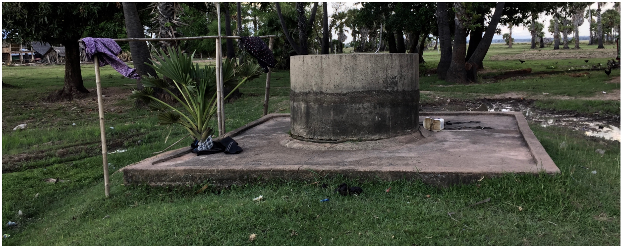
This well is a water source. There are feces on the ground beside it.
