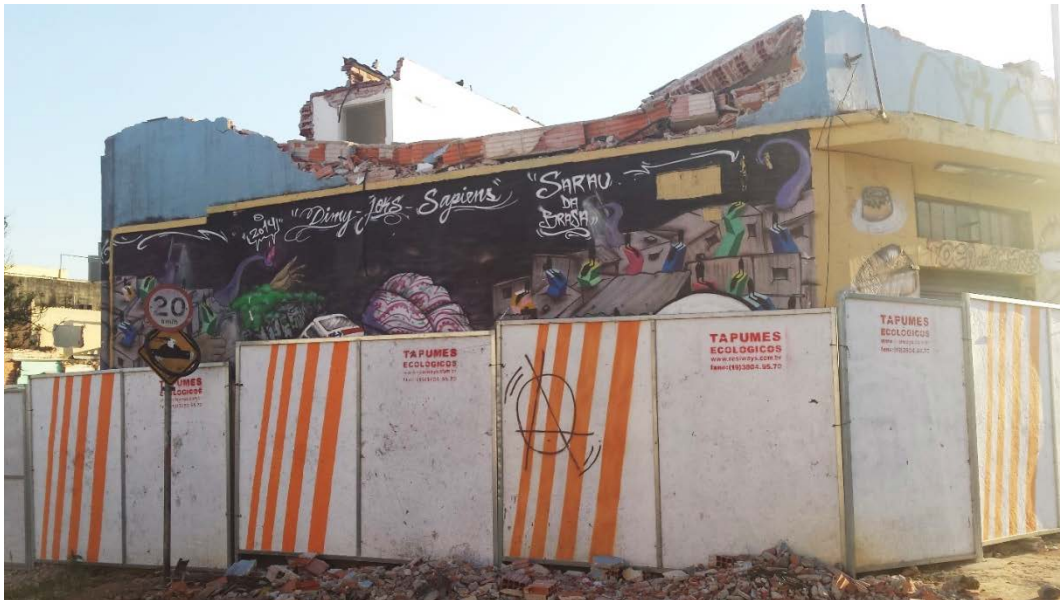
Figure 51: Construction partitions and half-demolished buildings in Brasília. Intersection of Estrada do Sabão and R. Prof. Viveiros Raposo. The building is now fully demolished. Photo by author, November 2016.
