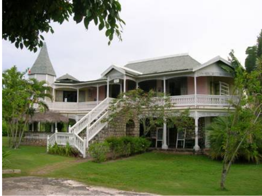
195. Harmony Hall, Tower Hill, St Mary (photographed in 2006)
