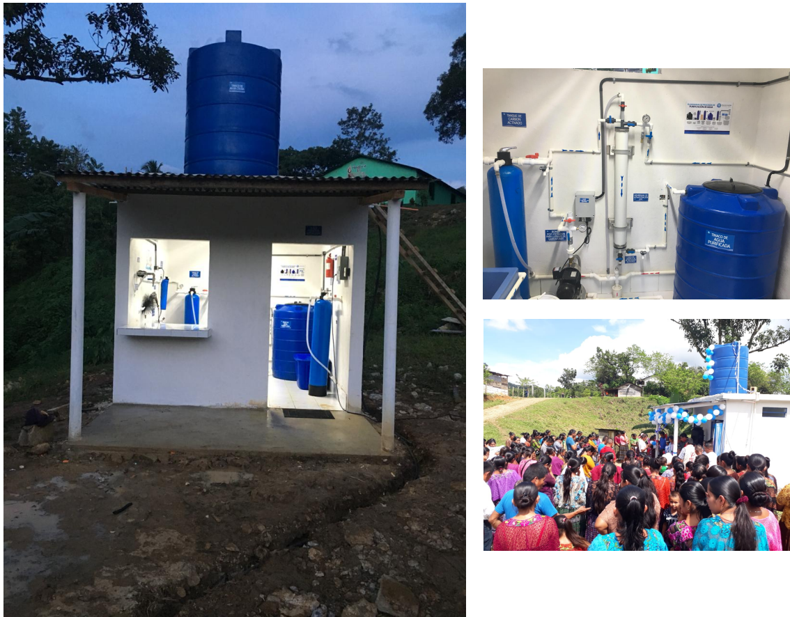
Figure 2. Photo of the completed water store (left) and the water purification system installed in the Sesajab community (top right). Photo of the inauguration of the water store in Sesajab with the community members in attendance (bottom right).
