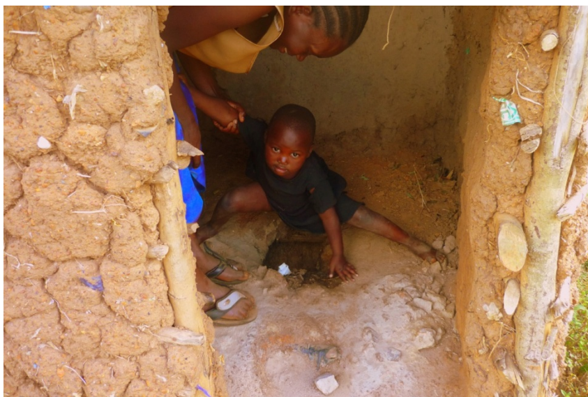
Figure 2 Child using a mud-floored pit latrine [5]
