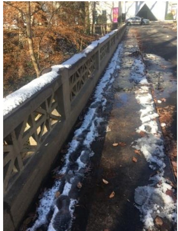
Figure 16. View of Mizell Bridge and Carlos Museum. Personal photograph by author.
