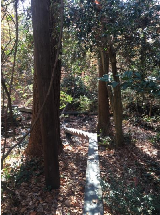
Figure 5. Last steel beam on northern slope. Personal photograph by author.
