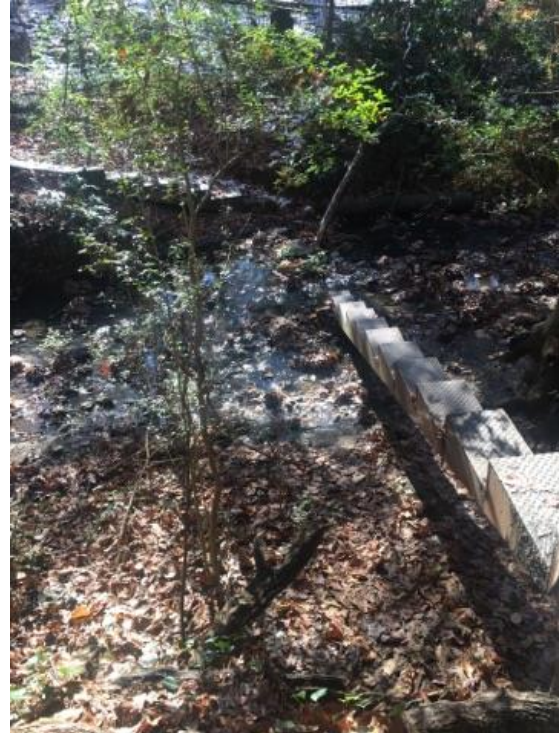
Figure 6. Suspended steel steps on northern slope. Personal photograph by author.
