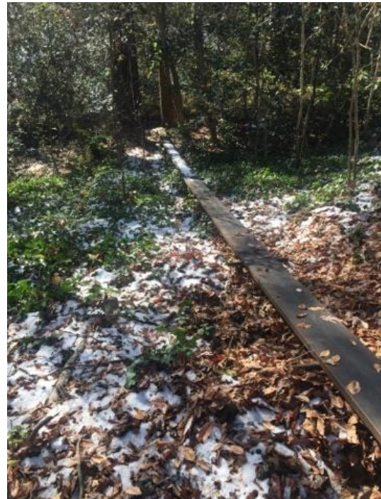
Figure 4. Center segment of series of steel beams on northern slope. Personal photograph by author.
