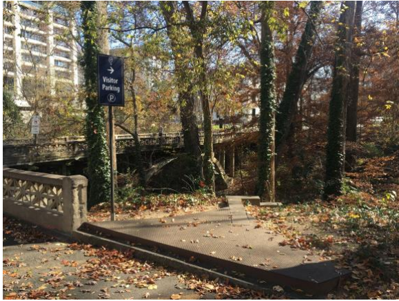
Figure 1. North entrance point of George Trakas's Source Route , 1979. Ferrous alloy, wood, concrete site-installation. 145.5 feet on south slope, 119.5 feet on north slope. Peavine Creek ravine, Baker Woodlands, Emory University, Atlanta, Georgia; Gift from Phi Beta Kappa, 1978. Personal photograph by author.
