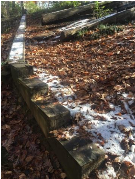
Figure 11. Wood steps connected to series of wood beams on southern slope. Personal photograph by author.
