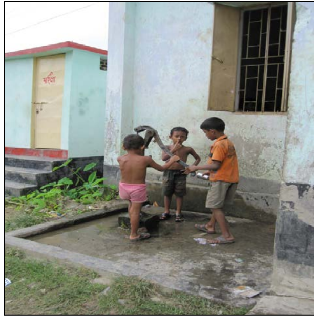
Figure 1.3 Typical school water source (tube well)
