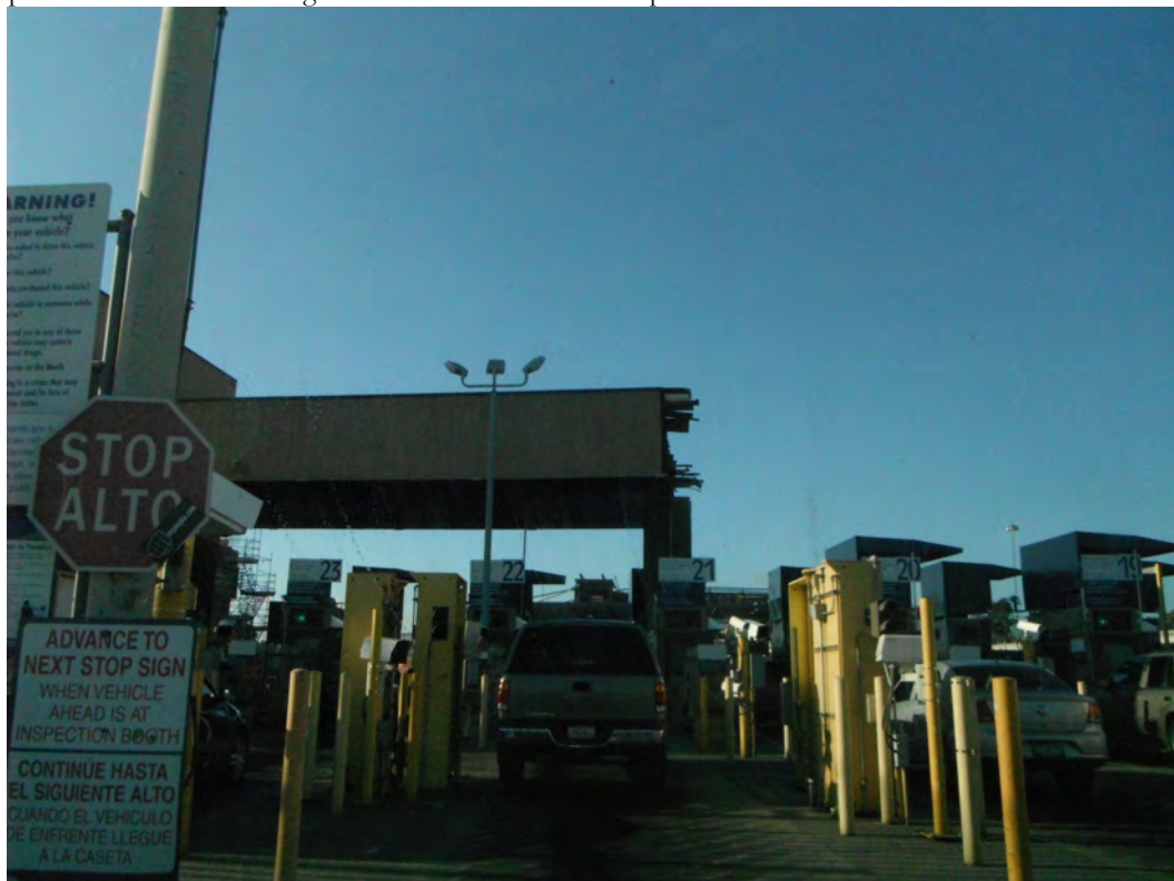
A view of the inspection booths under renovation in 2014...or of the fallen Linea ?
