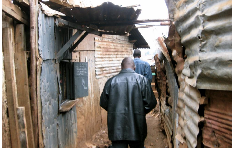
Figure 2: The width of the footpaths is often no more than that of one person, and pieces of metal are protruding from the structures
