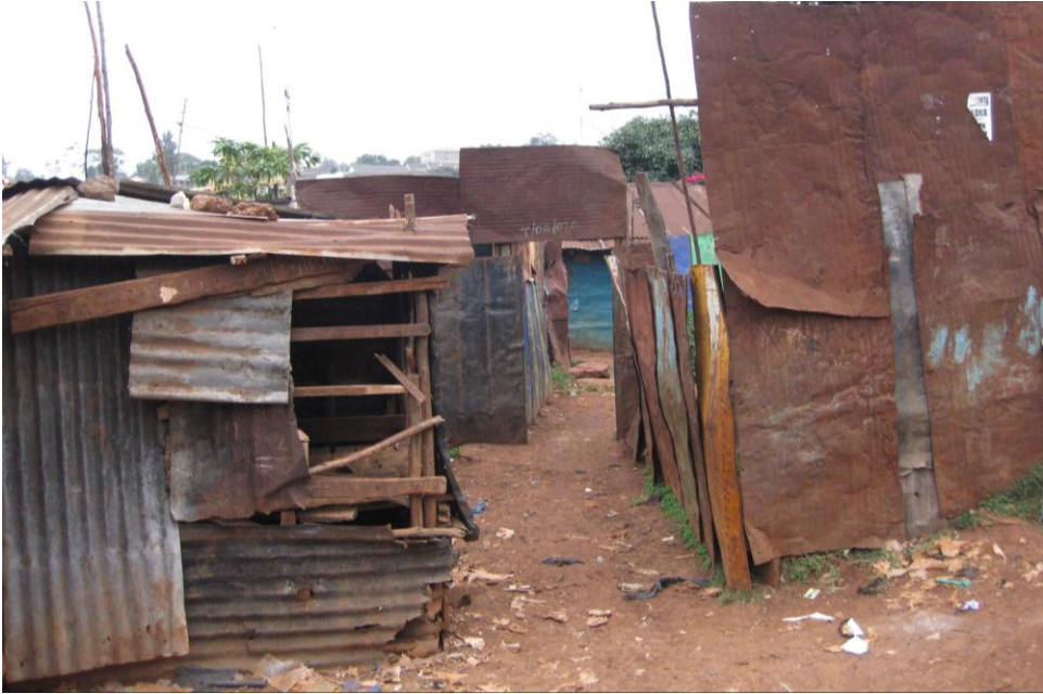
Figure 3: Example of construction materials and conditions of homes
